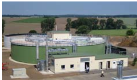
Dry Cycle Fermenter: Circular Plug Flow Anaerobic Digestion
